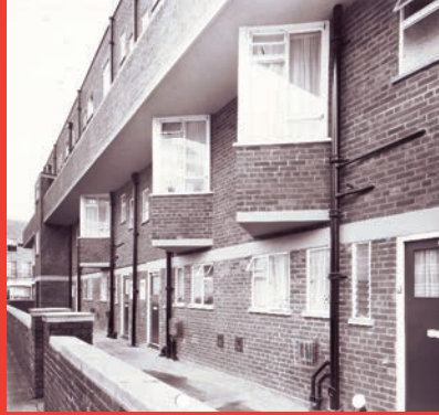
Refurbishment Works, Chelsea Manor Buildings, Chelsea
