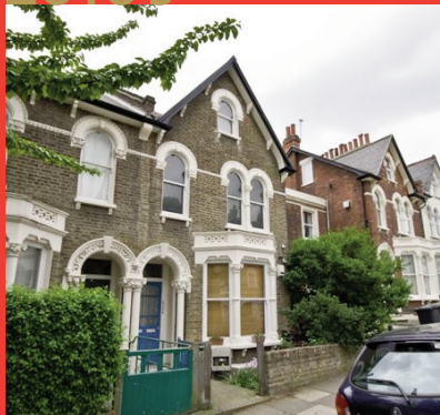
Refurbishment Works, Brockley PFI
